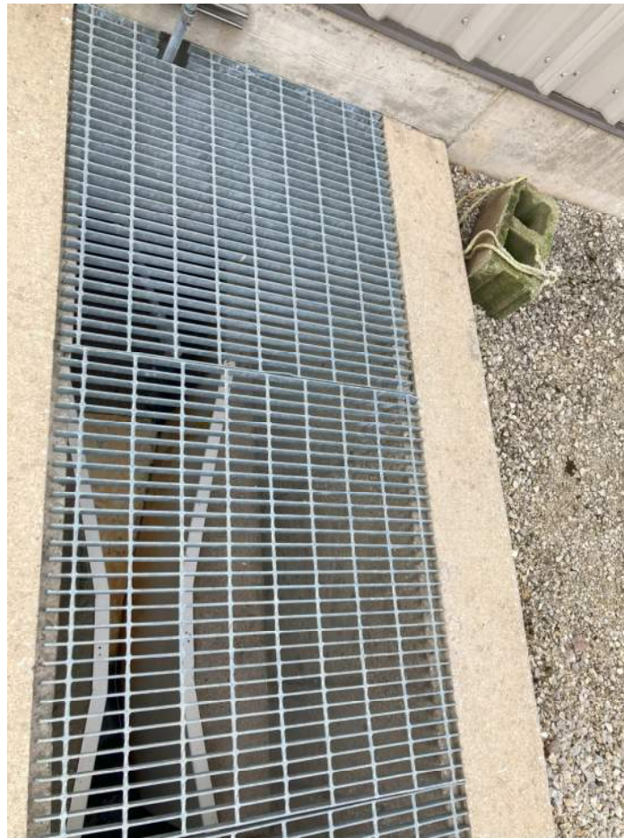
Figure 5: Photo indicating that the cinder block and attached rope have been removed from the Parshall flume
